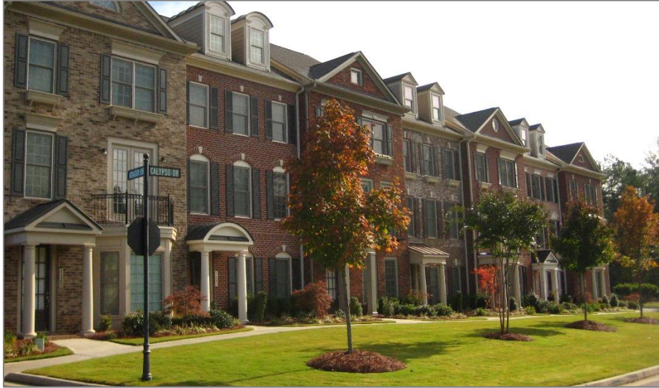
Figure 5.7.D(5)a: Changes in Building Façade
